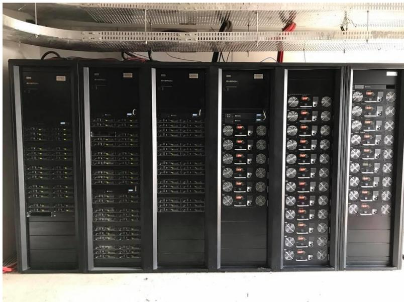
Figure 4: The EXERON system as an example of energy conversion units
