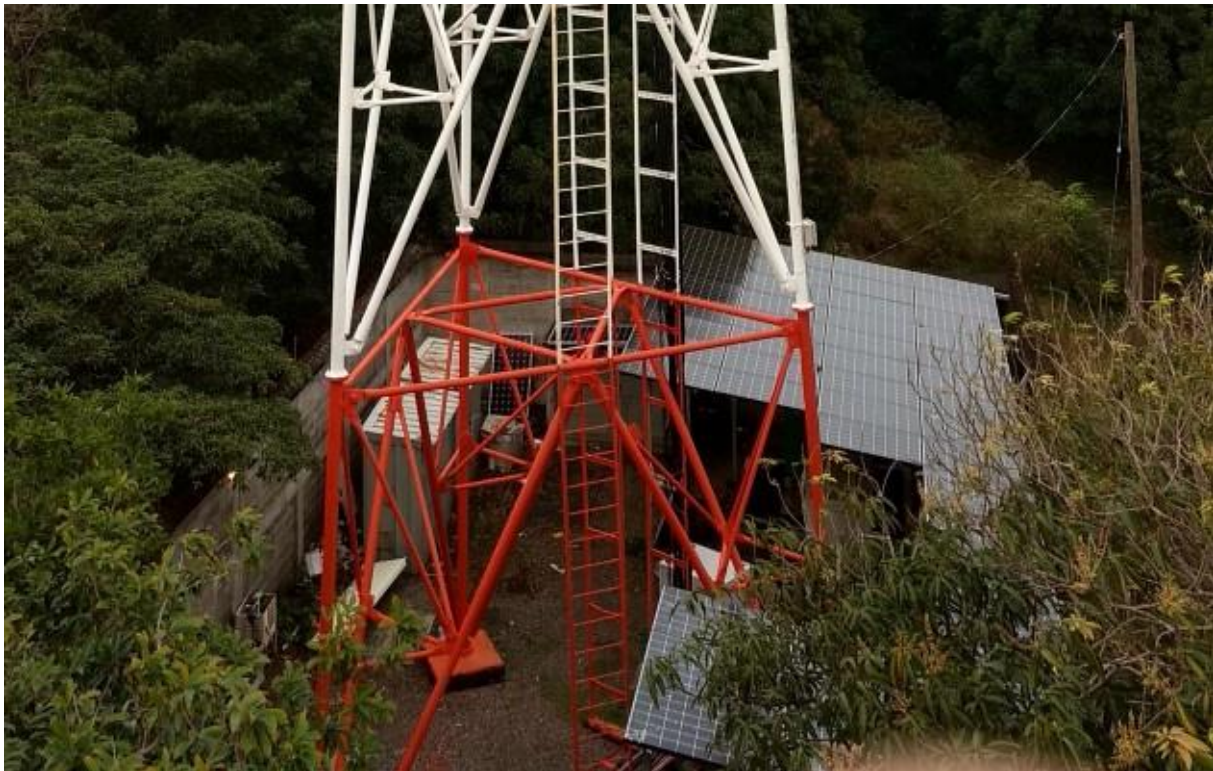
Figure 2: A solar array at a telecom tower at a remote island in Nicaragua
